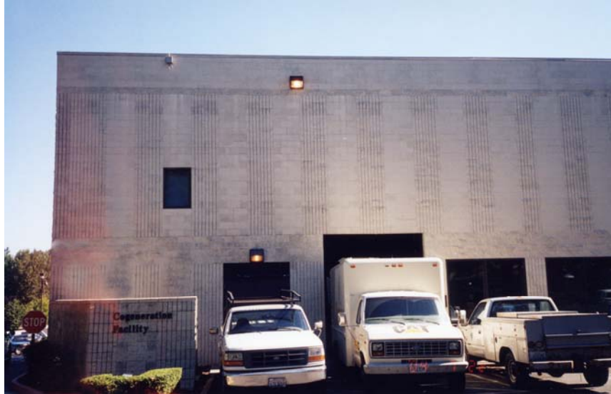
Figure 2. Cogeneration Plant at Valley Medical Center
