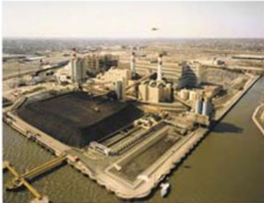
Eddystone Power Station (PA)- twin coal-fired units (combined 650MW) built in 1959 and still operating in 2007
