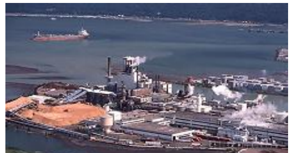
Aerial view of the Simpson Tacoma Kraft Mill
