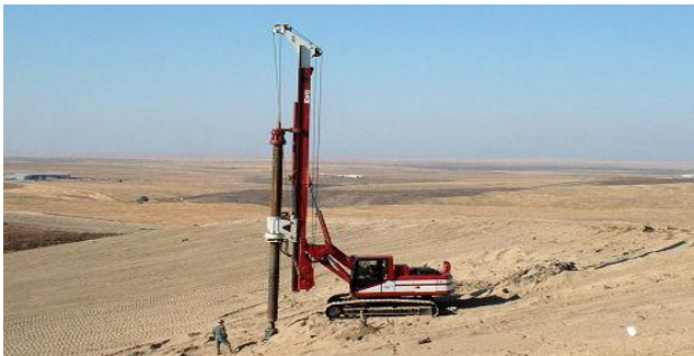
Installing vertical well
