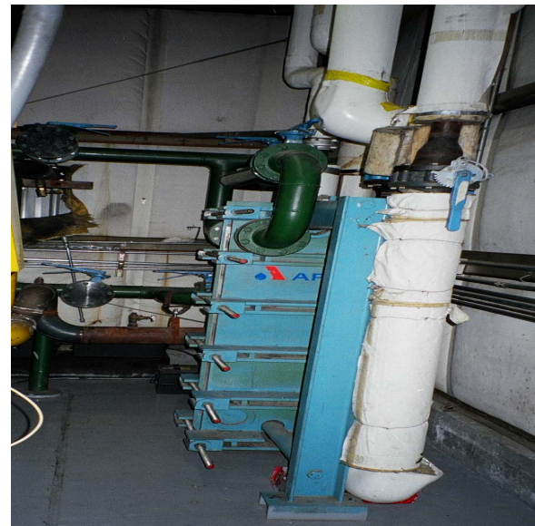
Figure 3: Recovered Heat System
